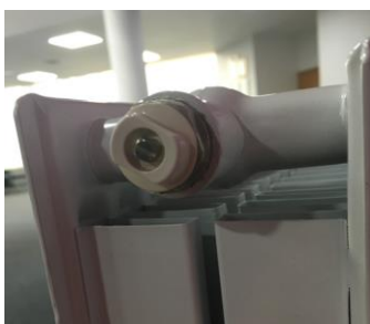
Radiator release valve
